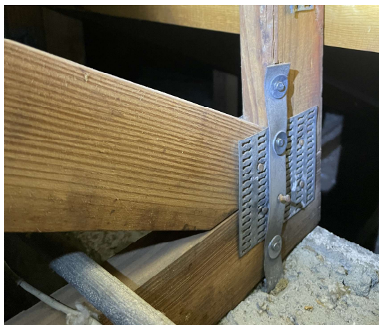
Roof to wall attachment - Clips
