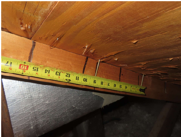
Roof deck nail spacing - Field
