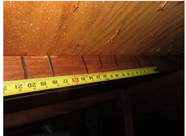
Roof deck nail spacing - Edge
