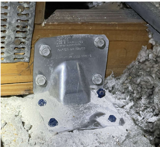
Roof to wall attachment - Clips
