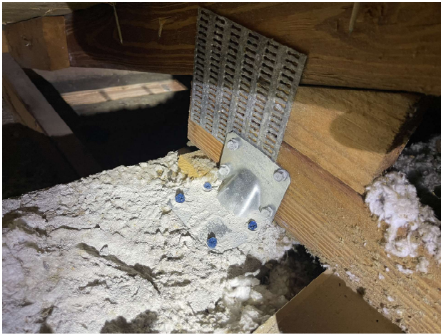
Roof to wall attachment - Clips
