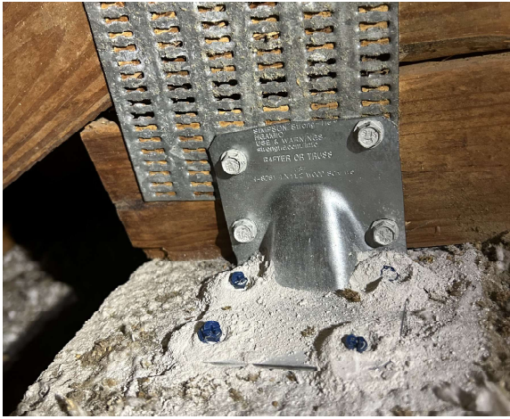
Roof to wall attachment - Clips
