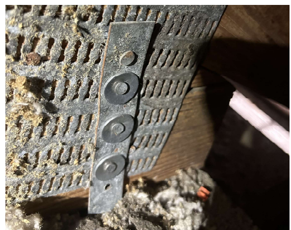
Roof to wall attachment - Clips
